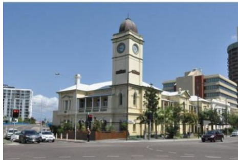
Figure SC6.3.5.32 Illustrates a desirable outcome: former Post Office building (Flinders Street, Townsville)
